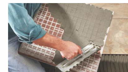
2. Cement laying on Tile
