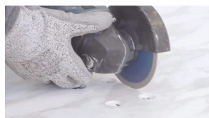
2. Cut with Diamond Blade Angle Grinder
