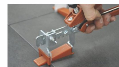
4. Levelling Wedges
