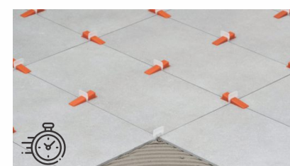
5. After Levelling Process leave it for 8-10 hrs.
