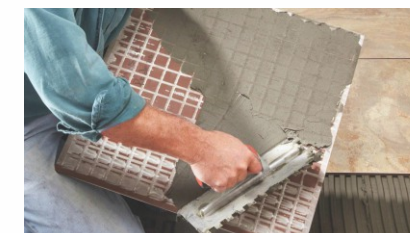
2. Cement laying on Tile
