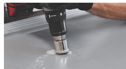
1. Round Cut with Diamond Blade Drill
