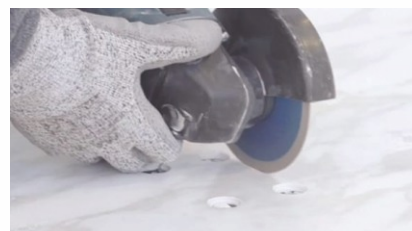
2. Cut with Diamond Blade Angle Grinder
