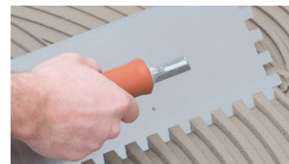
1. Cement laying on Floor
