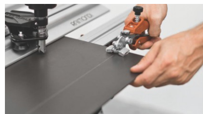
2. Cutting of Tile
