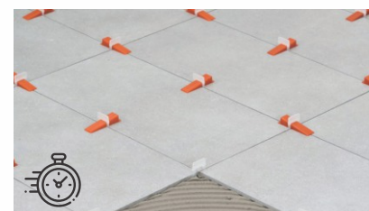
5. After Levelling Process leave it for 8-10 hrs.
