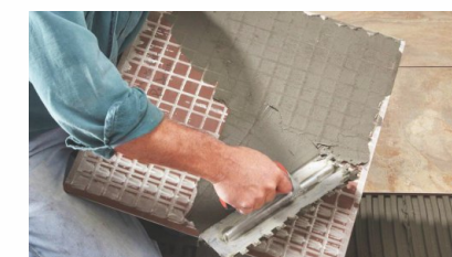
2. Cement laying on Tile
