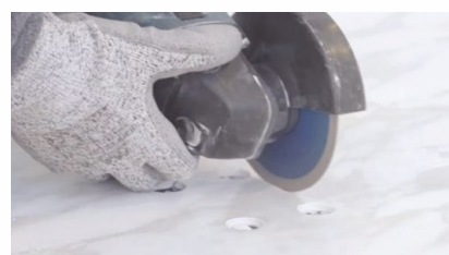
2. Cut with Diamond Blade Angle Grinder
