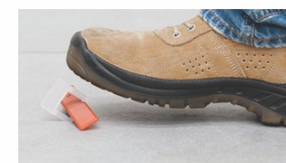
6. Remove Wedges ones it Dry
