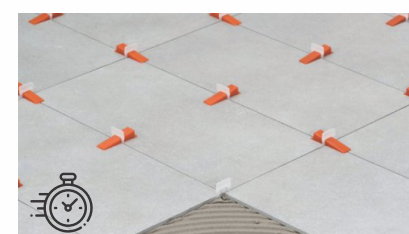
5. After Levelling Process leave it for 8-10 hrs.
